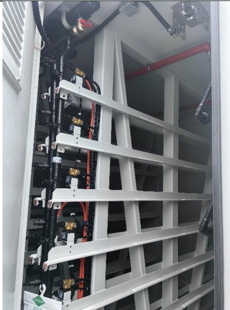
Battery cabinet without battery pack equipped
