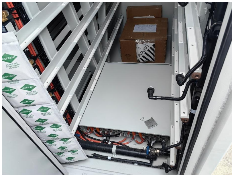
Battery cabinet without battery pack equipped
